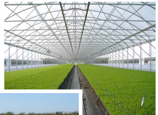
18' x 408' T-Rail bench in a 40' wide Thermolator.
