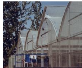
Insulator with inflatable tropical vent for mild climates.
