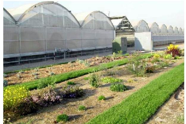
Insulator production houses with conveyer system feeding into a head house.
