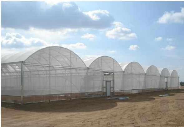
Insulator used as a screen house to protect citrus trees from the psyllid bug.
