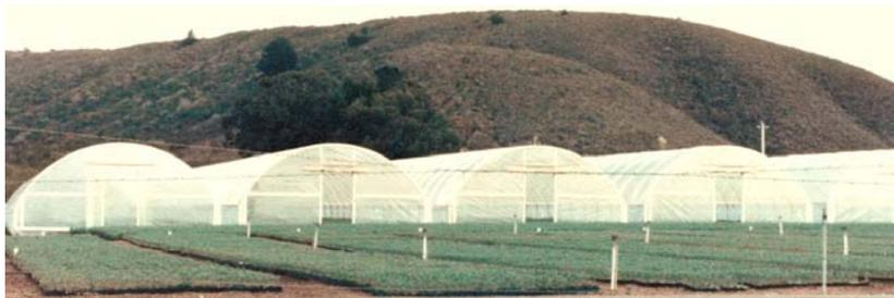
Cold frame 20's with poly roof with Agra Tech' standard endwall options designed for corrugated polycarbonate.
