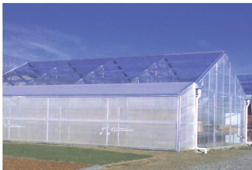
Lean-To Screen house over Pad Vent.
