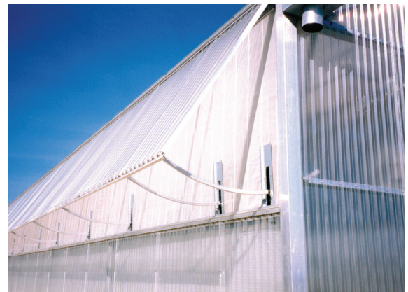
Insect screen installed with a wall-vent.
