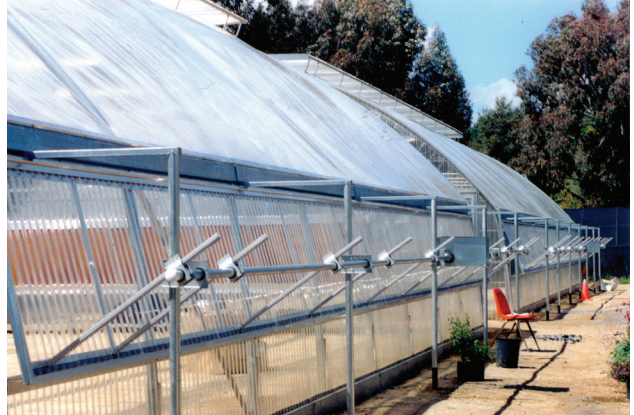
Peak Vent in Poly Roof & Pad Vent
