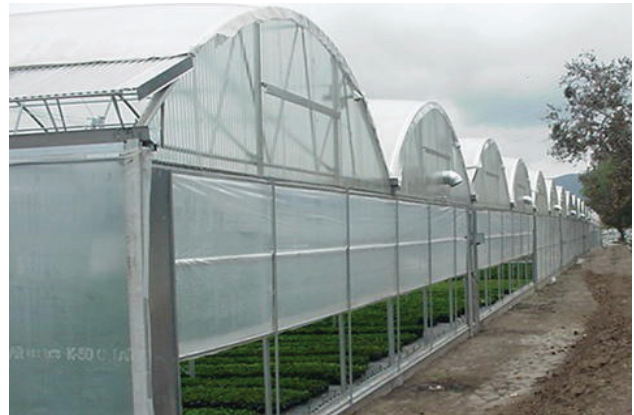
Gutter Vent in Poly Roof & Roll Up Wall
